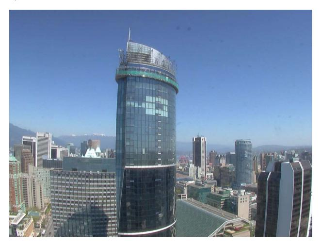
Work on the 48<sup>th</sup> floor is complete, the stage is being lowered to the 47<sup>th</sup> floor at this moment (you can see the dark glass emerging above the suspended work platform). We are pushing to have work complete on the 47<sup>th</sup> floor by Friday the 17<sup>th</sup>, then on to our one floor/week target.
