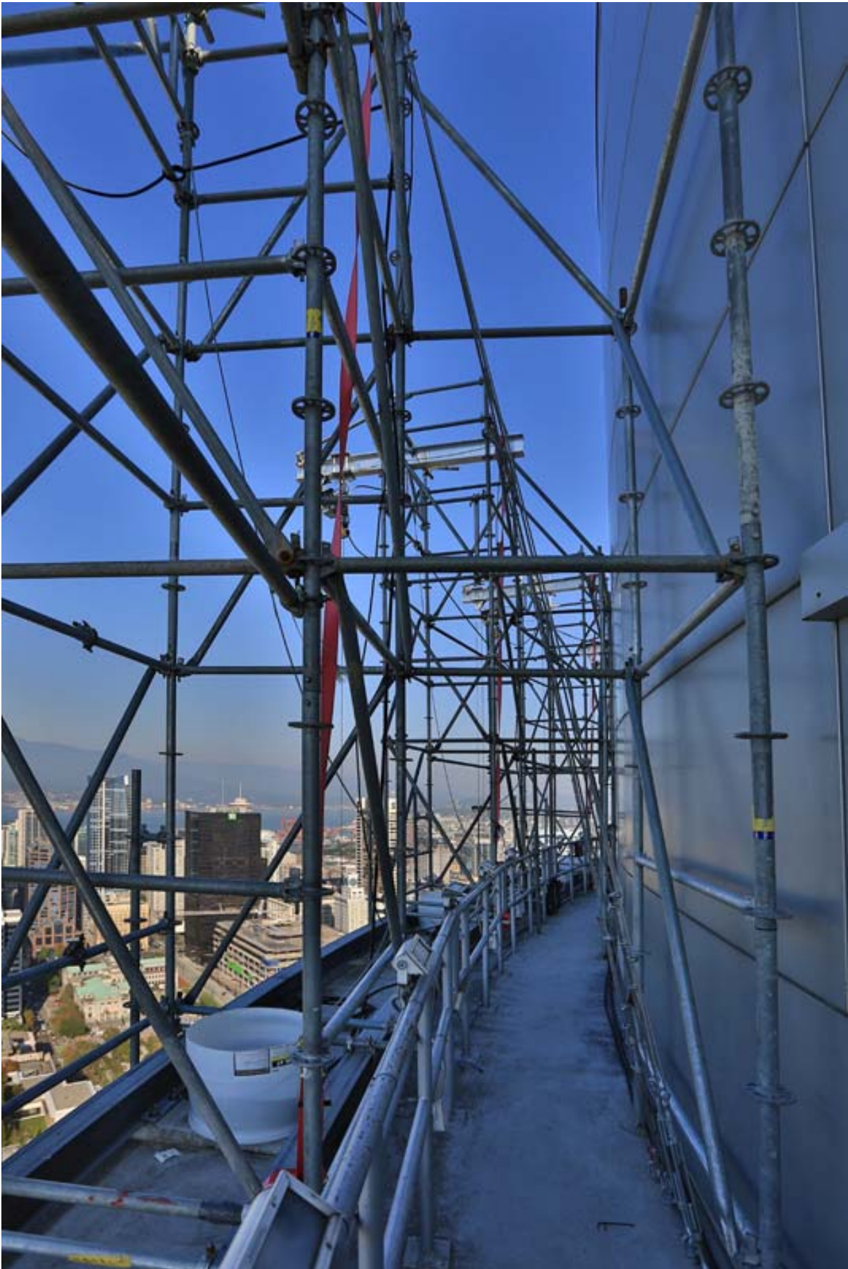
Views of the roof top scaffolding and support structures for the platform
