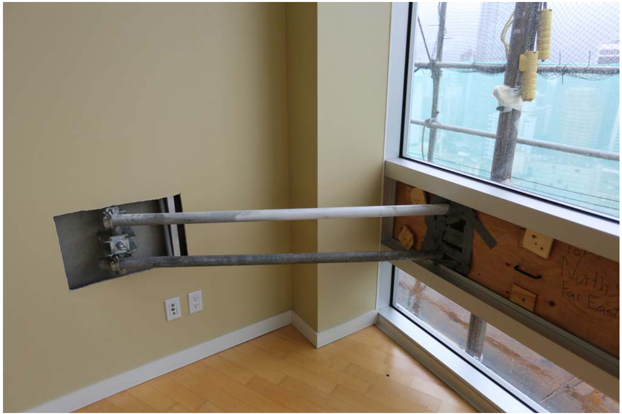
Platform anchor to bedroom wall
