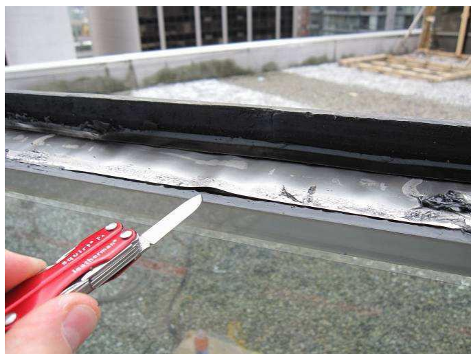
Fig. 3.7.1.3 Typical ripple or "fish mouth" in the stainless steel edge band of IGU 43161
