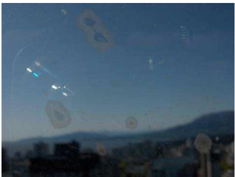
Large low-e corrosion spots visible from 3m
