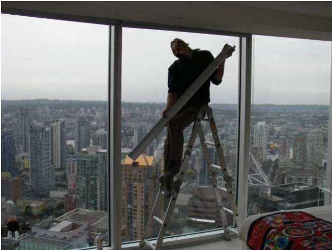
Figure B6: Removal of curtainwall framing component to access desiccant tube to attachment of pressure gauge tubing
