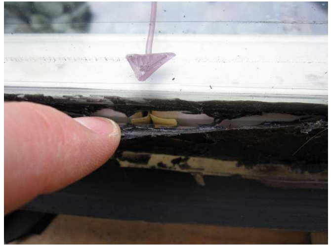
Fig. 3.7.1.6 Typical delamination of the stainless steel edge band at a large joint in the PVC spacer between the jamb and corner of IGU 43161.
