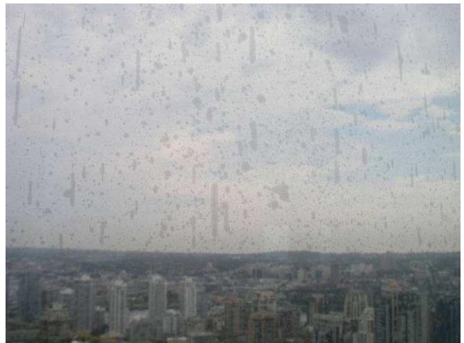
Figure F38: Suite 3903, July 3, 2008, low-e corrosion on glass surface #2.
