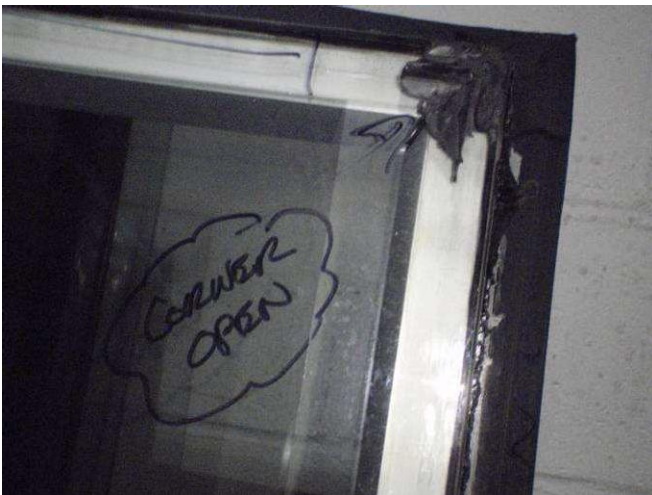
Figure E84: Stainless steel edge band discontinuity #9, at corner.
