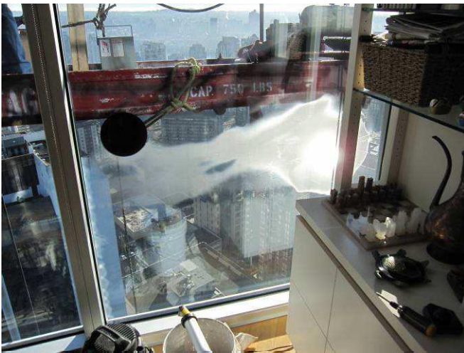
Figure E18: Interstitial fogging within IGU 44789, as result of shading of swing-stage on unit. IGU heated by sunlight to drive moisture out of desiccant resulted in condensation of moisture on colder shaded surface.
