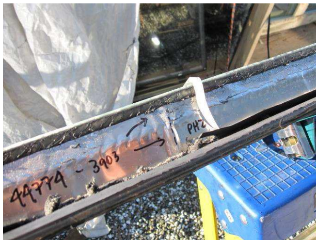
Figure E4: Buckling of stainless steel edge band (edge seal discontinuity PH2). See Figure E76 for edge seal drawing.
