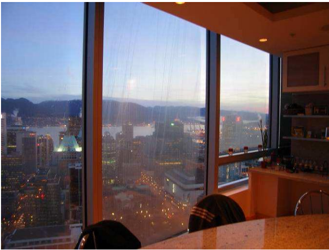
Figure F25: Suite 4702, January 24, 2006, fogged/frosted IGUs.
