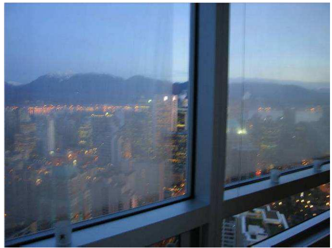
Figure F22: Suite 4702, January 24, 2006, fogged/frosted IGUs.
