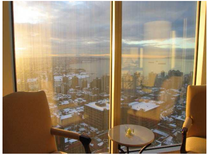
Figure F20: Suite 4702, January 9, 2005, fogged/frosted IGUs.
