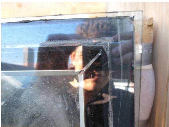
Figure E3: Corner condition of IGU 44774.
