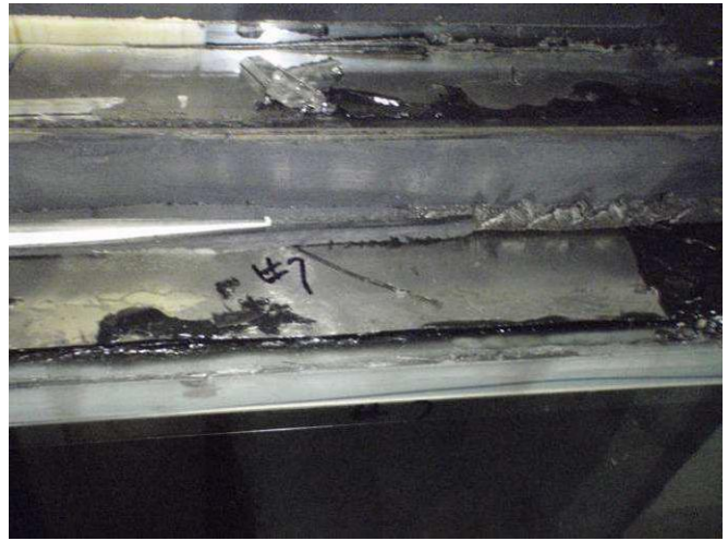
Figure E81: Stainless steel edge band discontinuity #7
