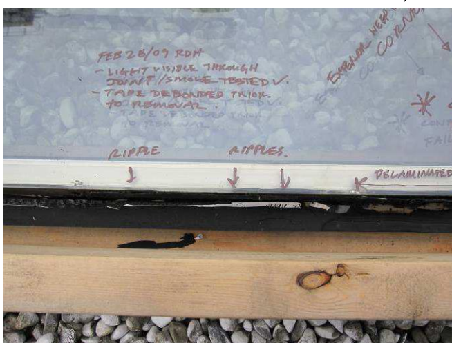
Figure E37: Discontinuities in edge seal noted at left jamb of IGU.
