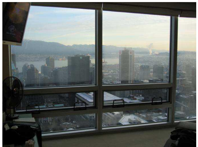
Figure F30: Suite 4602, January 14, 2007, fogged/frosted IGUs.
