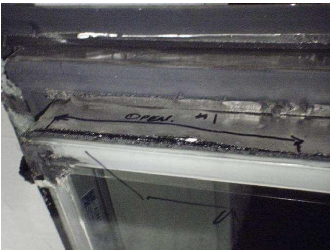
Figure E70: Stainless steel edge band discontinuity #1 at corner of unit, allowing for air-leakage into IGU at vinyl corner/vinyl jamb extrusion joint. See Figure E98 for an edge seal schematic.
