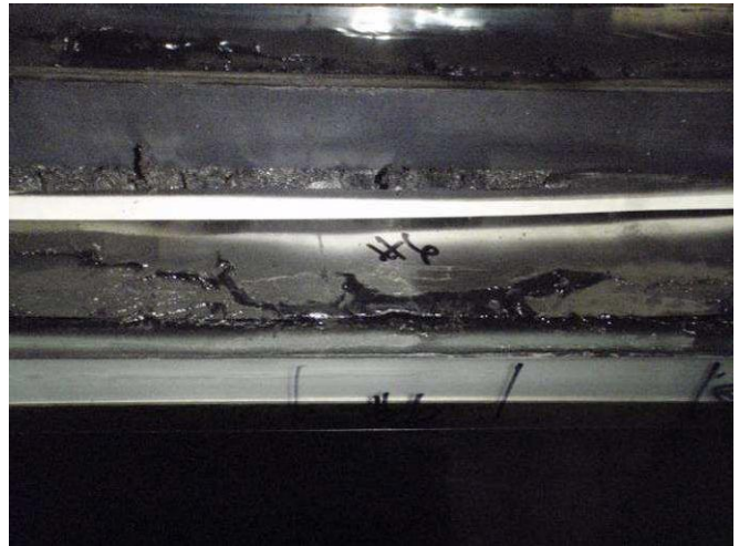
Figure E79: Stainless steel edge band discontinuity #6.
