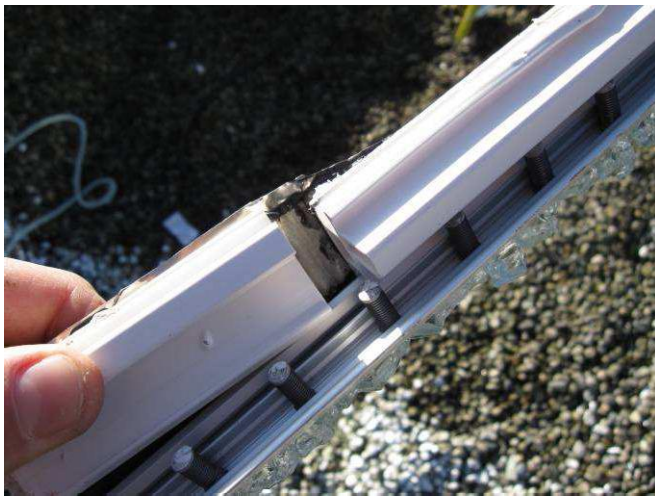
Figure E14: Vinyl extrusion edge spacer, note gap between components.
