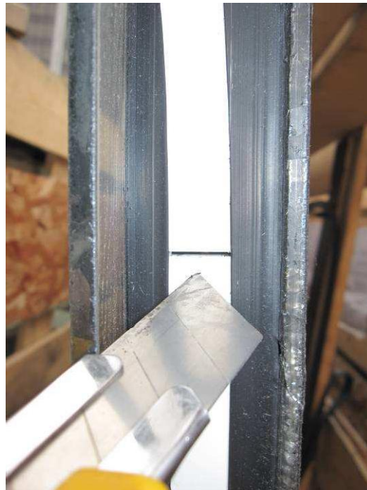
Figure E95: Joint between vinyl extrusions – allows airflow directly into IGU if stainless steel foil is compromised.
