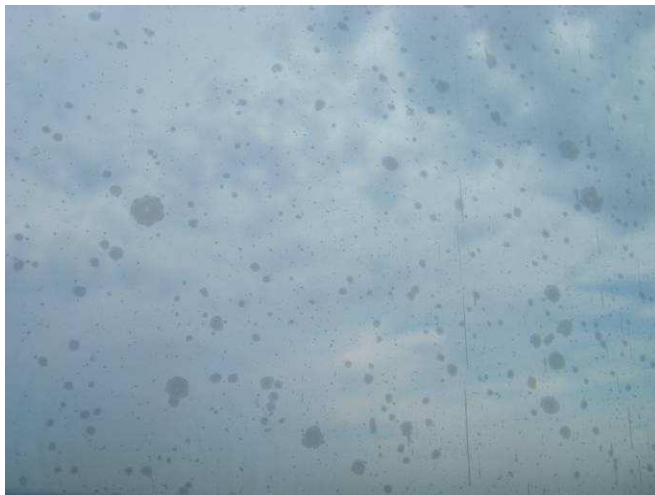
Figure F37: Suite 3903, July 3, 2008, low-e corrosion on glass surface #2.
