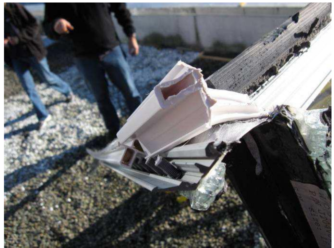
Figure E15: Typical corner configuration with welded vinyl corner piece. Long extrusion along sill and jambs is not connected to the corner piece, a significant discontinuity and therefore relies on stainless steel foil to be air-tight.
