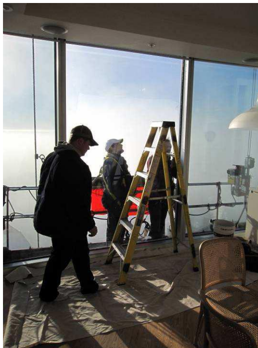
Figure E2: Removal of IGU using crane and swing stage
