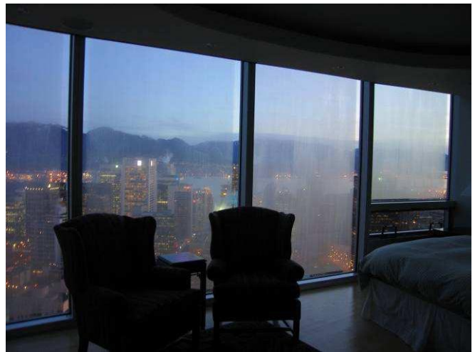
Figure F24: Suite 4702, January 24, 2006, fogged/frosted IGUs.
