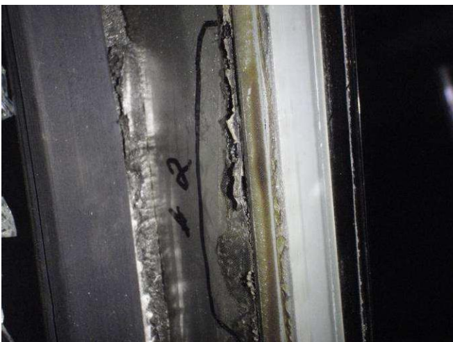
Figure E72: Stainless steel edge band discontinuity #2.
