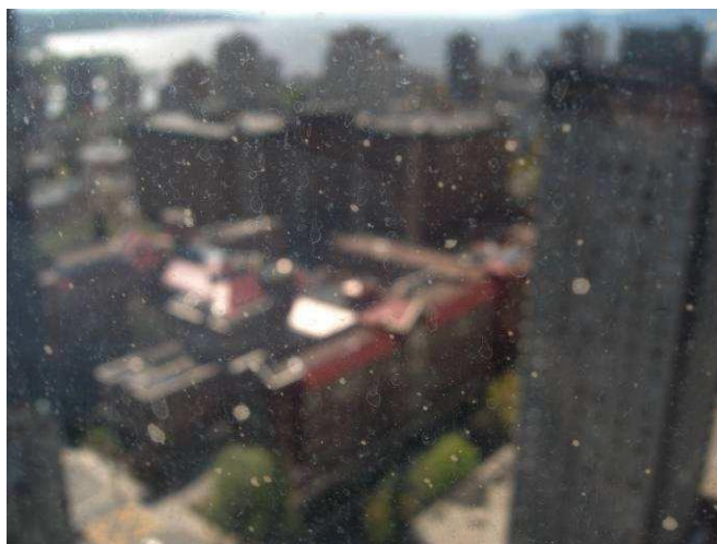
Figure F33: Suite 3101, May 15, 2008, low-e corrosion spots on glass surface #2.
