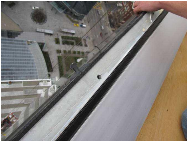
Figure E24: Sill of glazing pocket, clean and dry. Drainage hole at center shown, additional drainage holes at each jamb.
