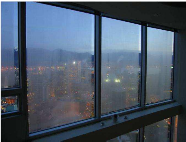
Figure F21: Suite 4702, January 24, 2006, fogged/frosted IGUs.
