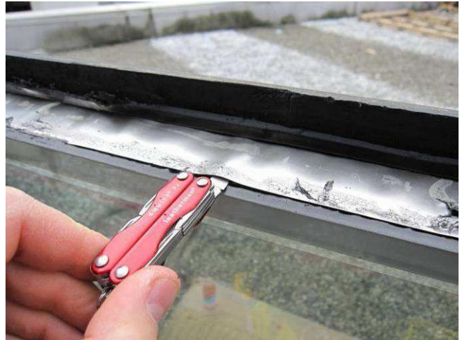
Figure E32: Foil ripple edge seal discontinuity shown in Figure E31.
