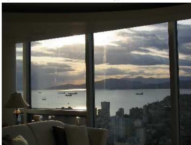
Figure F4: Suite 4702, July 7, 2004, fogged/corroded IGUs.
