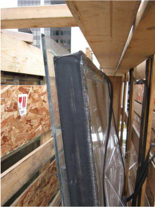
Figure E92: Broken “new” style of Vision Wall IGU with alternate perimeter edge seal. Edge seal band was disassembled to determine as-built and air-sealing details. See Figure E99 for drawing.
