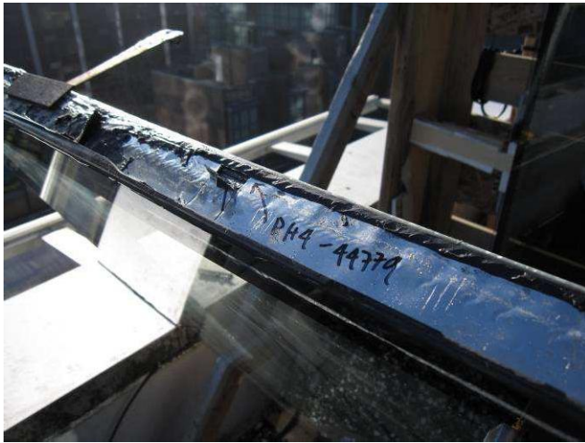
Figure E10: Buckling of stainless steel edge band (edge seal discontinuity PH4).
