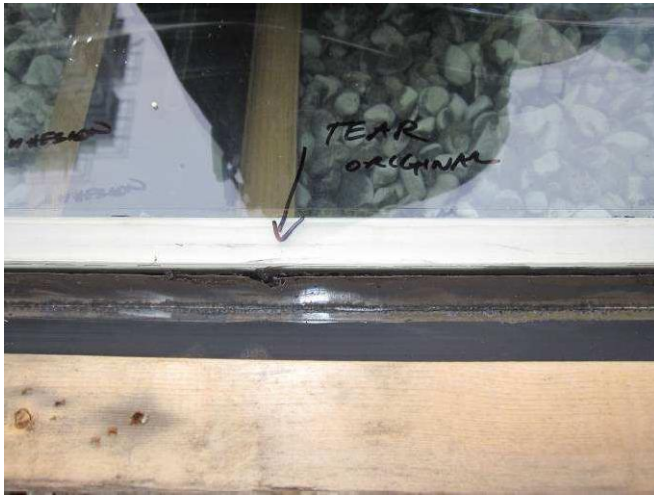
Figure E39: Tear in stainless steel edge band noted at sill.
