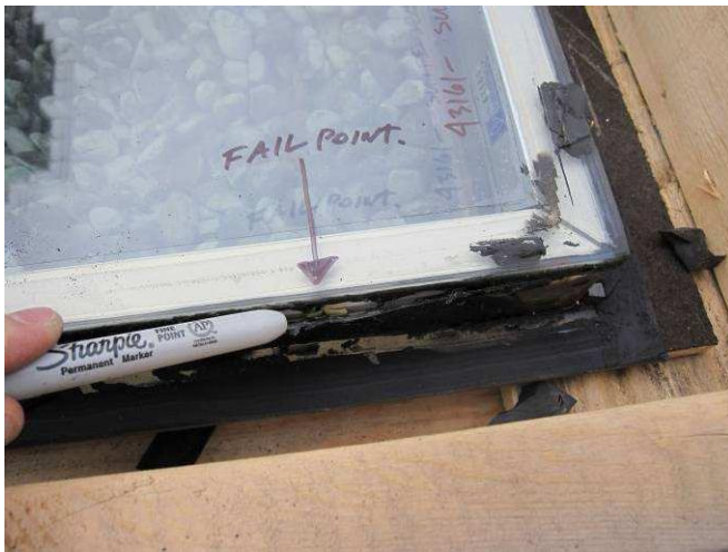
Figure E33: Location of large discontinuity in stainless steel edge seal. Delamination of stainless seal air-seal at the open joint between the vinyl corner and jamb spacer extrusion.
