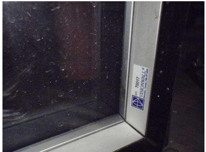
Figure E89: Suite 3803 Replacement IGU 70017, in parking garage – severe low-e corrosion already noted.
