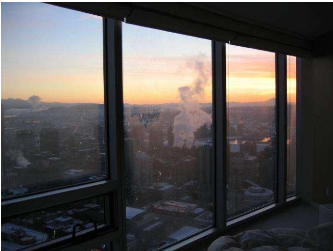
Figure F27: Suite 4602, January 14, 2007, fogged/frosted IGUs.
