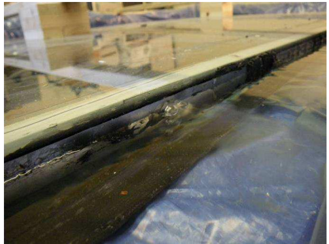
Figure E47: Edge seal discontinuity #15.
