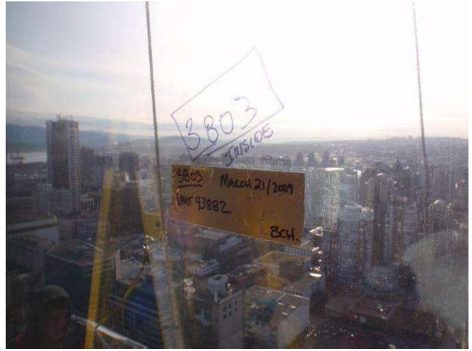
Figure E65: IGU 43882 prior to removal, severe low-e corrosion on IGU surface #2.
