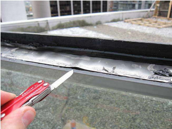
Figure E31: One of many fish mouth discontinuities in perimeter stainless steel foil edge seal.
