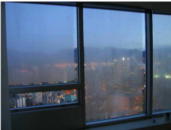
Figure F23: Suite 4702, January 24, 2006, fogged/frosted IGUs.
