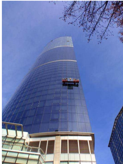
Figure E67: Removal of IGU 43882 from suite 3803 at southeast corner of building.
