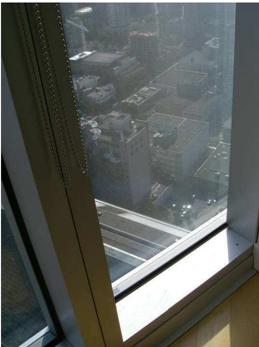
Figure F41: Suite 3903, IGU 45484, August 7, 2008, low-e corrosion on glass surface #2.
