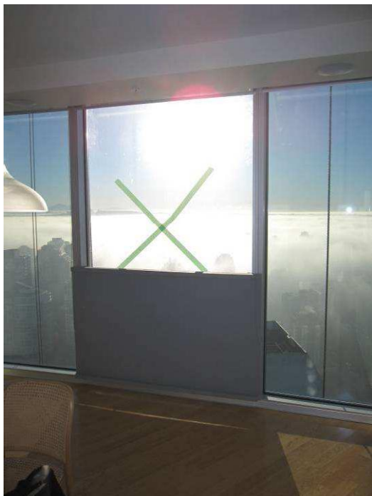
Figure E1: IGU 44774, Suite 3903 to be removed. Inner lite of tempered glass broke in October 2007 as the result of a nickel sulphide glass inclusion.
