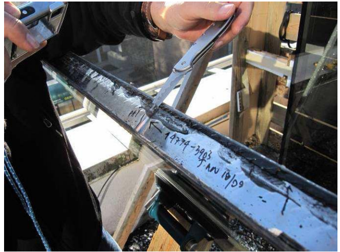
Figure E6: Buckling of stainless steel edge band (edge seal discontinuity PH1). Knife inserted into fish-mouth to show un-adhered edge seal.
