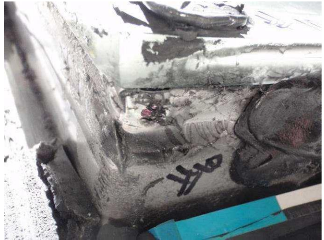
Figure E87: Stainless steel edge band discontinuity #9 at corner.
