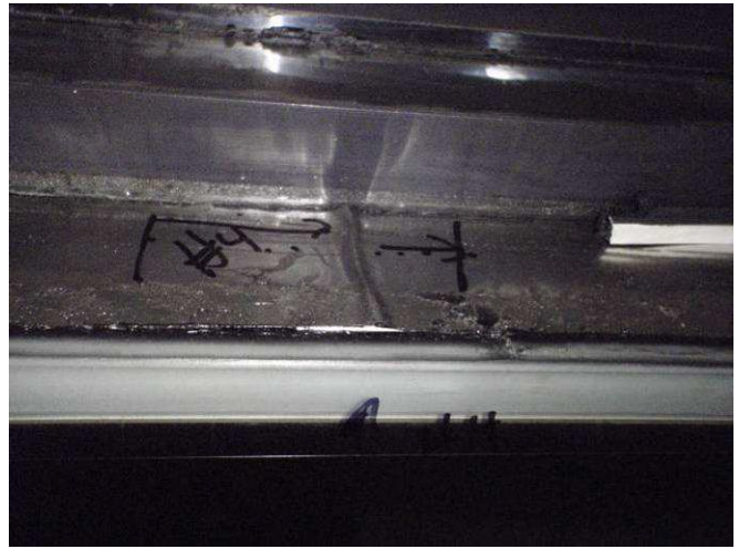
Figure E75: Stainless steel edge band discontinuity #4.
