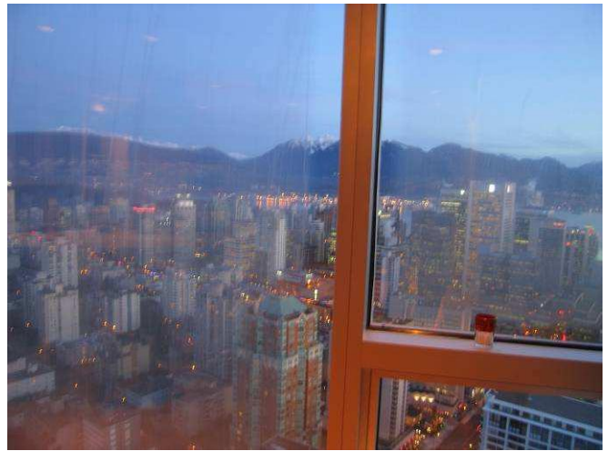
Figure F26: Suite 4702, January 24, 2006, fogged/frosted IGUs.
