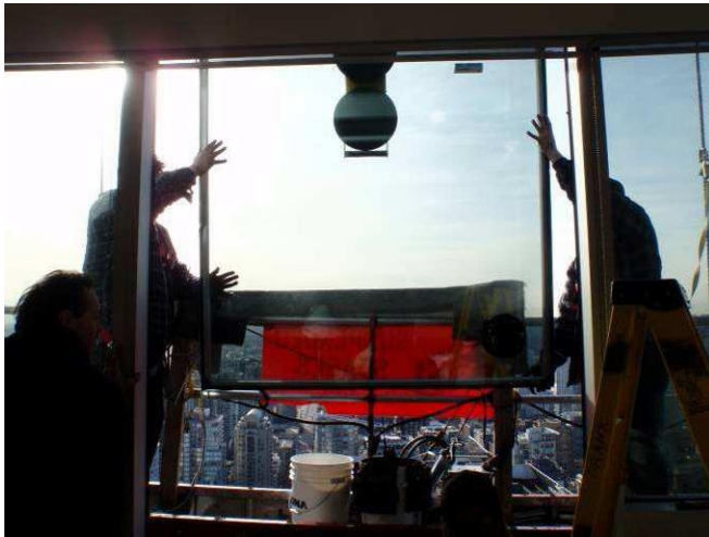
Figure E64: IGU 43882 removed from suite 3803, master bedroom – severe low-e corrosion noted.
