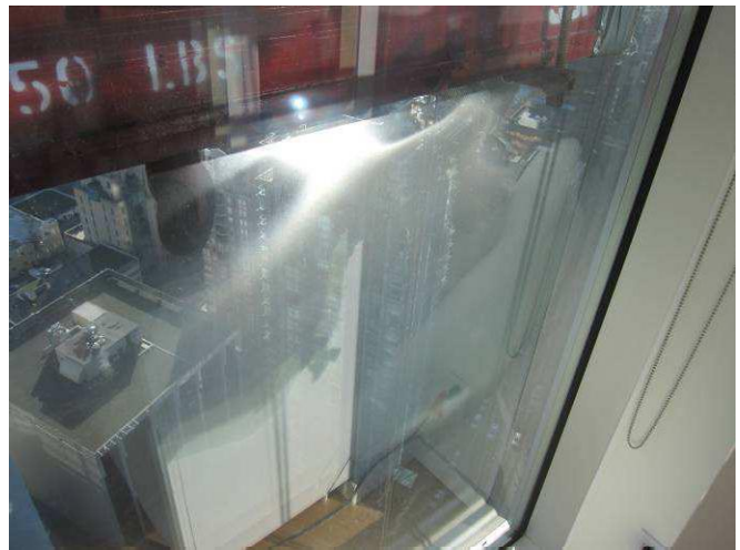
Figure E19: Interstitial fogging within IGU 44789, as result of shading of swing-stage on unit. IGU heated by sunlight to drive moisture out of desiccant resulted in condensation of moisture on cold shaded surface.
