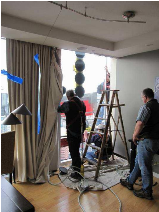
Figure E25: Removal of IGU from frame by contractor.
