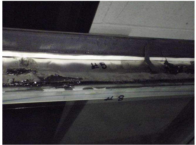
Figure E83: Stainless steel edge band discontinuity #8.
