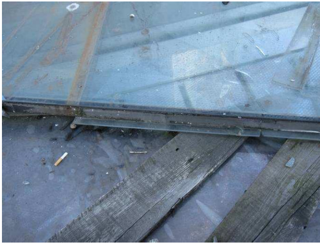
Figure E20: Old unmarked IGU on roof previously replaced by a contractor as result of tempered lite glass breakage. IGU edge condition reviewed during visit.
