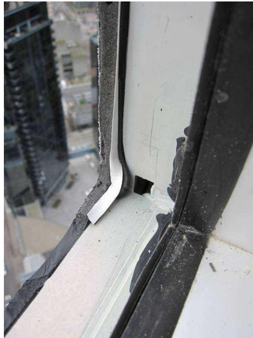
Figure E26: Sill corner drain hole into jamb. Drainage cavity clean and dry with no visible evidence of liquid water penetration.
