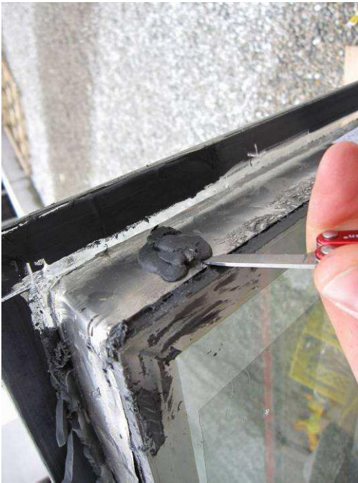
Figure E29: Location of desiccant tube – cut by contractor during glazing removal. The tube appeared well sealed into the IGU.
