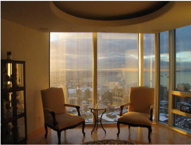
Figure F19: Suite 4702, January 9, 2005, fogged/frosted IGUs.
