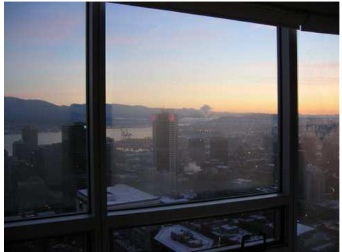
Figure F28: Suite 4602, January 14, 2007, fogged/frosted IGUs.
