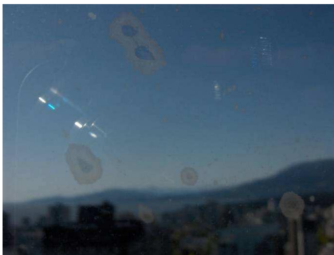
Figure F34: Suite 3101, May 15, 2008, low-e corrosion spots on glass surface #2.
