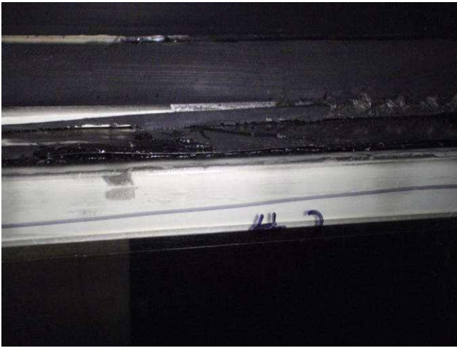
Figure E80: Stainless steel edge band discontinuity #7.
