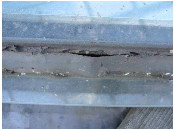
Figure E21: Unmarked IGU, one of several fish-mouth openings in stainless steel edge band – similar to that observed on removed unit 44774.
