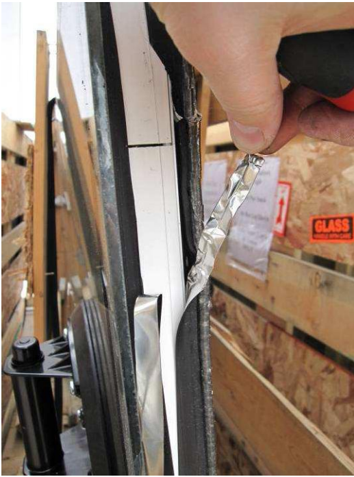
Figure E96: Edge of foil wrapped and sealed as shown in Figure E99.
